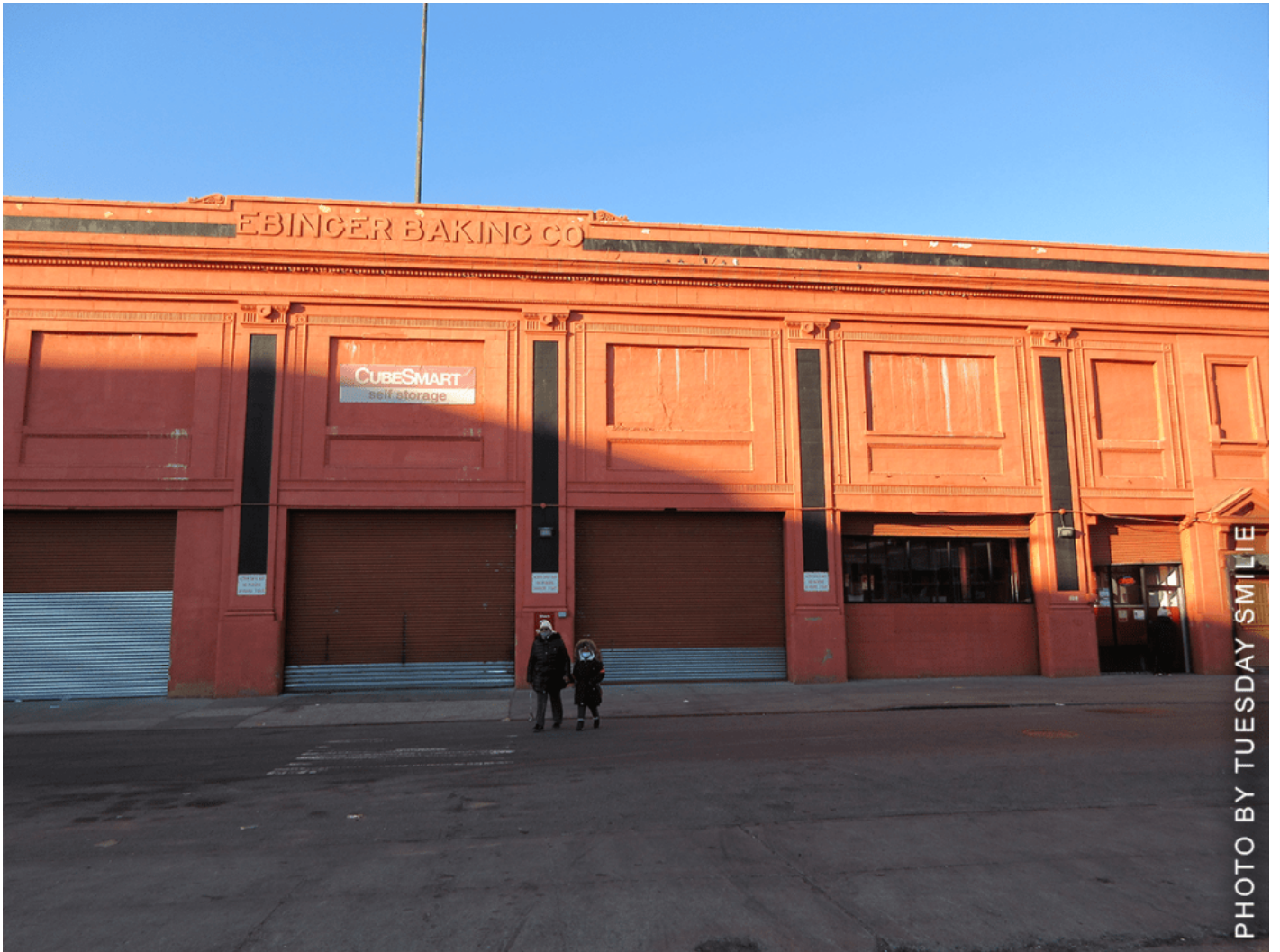
Ebinger Baking Company is long gone, but the their name is still present on the facade of the old truck depot.
