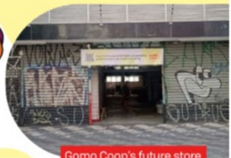
Gomo Coop's future store under construction
